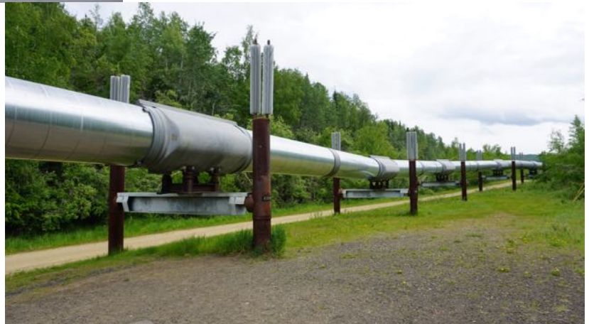
The pipeline north of Fairbanks
