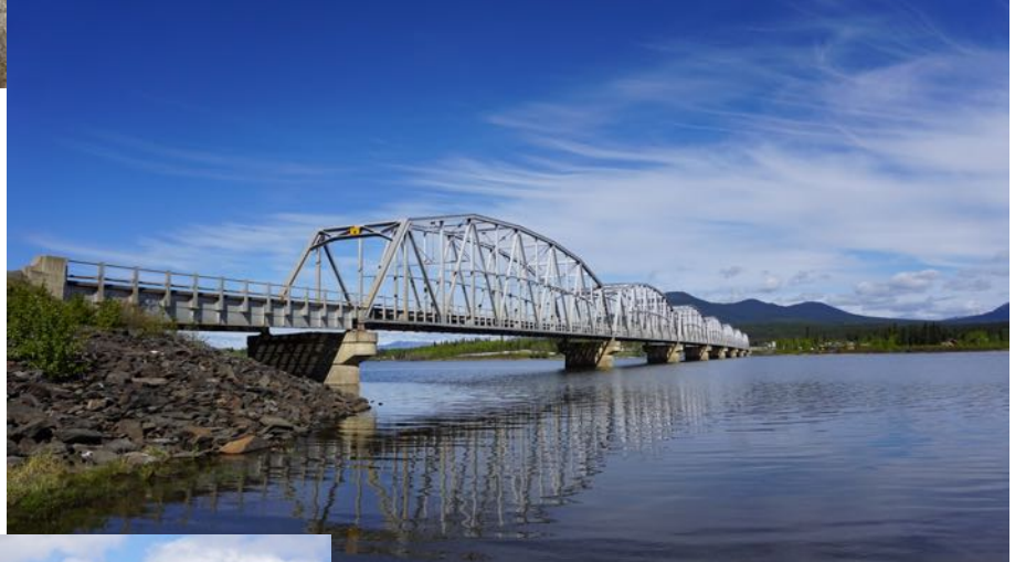
Bridge into Teslin, YK
